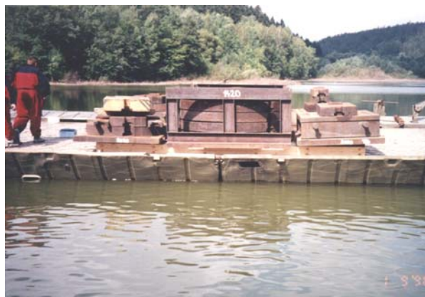
Fig. 15 – Experimental measurement on floating bridge PMS
