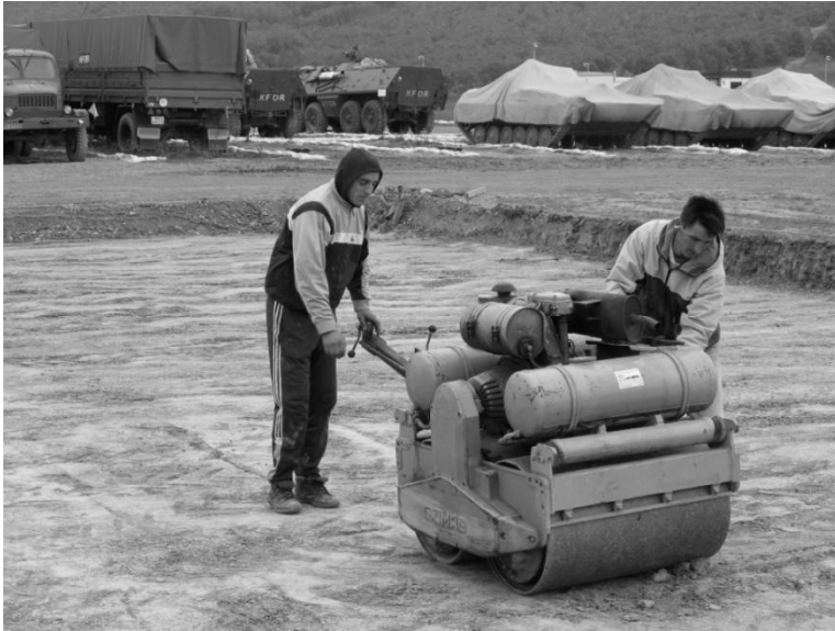
Fig. 1 Firming the subsoil
