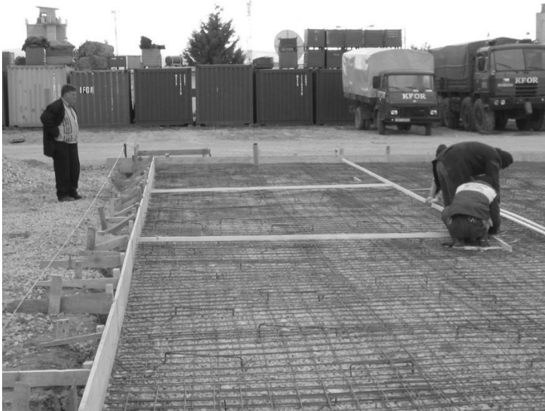
Fig. 2 Laying the KARI meshes
