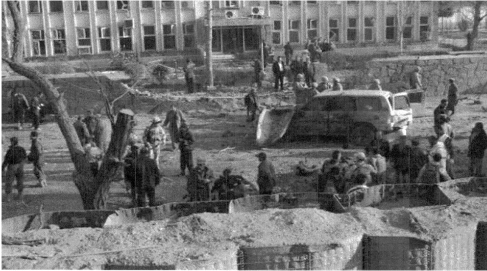
Fig. 5 Comparison of damages on rigid and loose protection structures (archive of the author)
