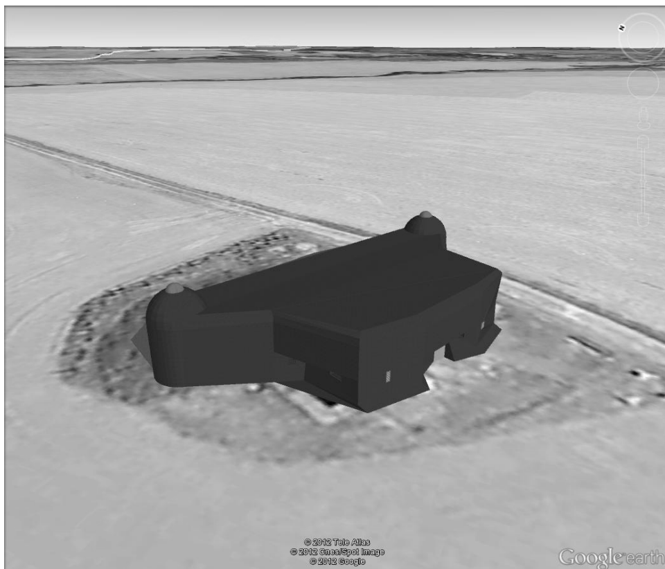
Fig. 12 A 3D Model of the infantry blockhouse OP – S 25 in the application Google Earth
